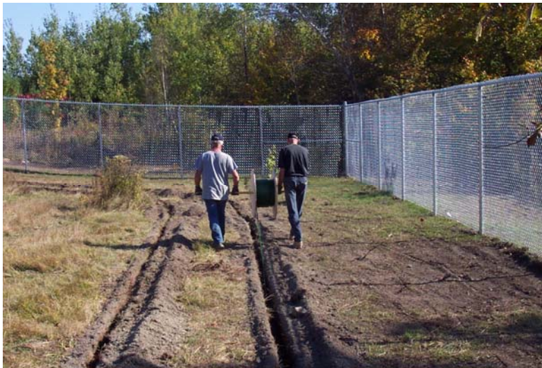
Figure 6.3 – Installing Sensor Cable in Soil
